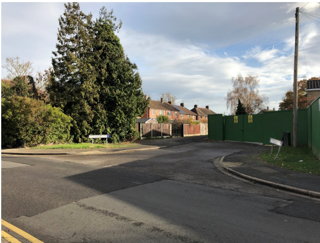
Existing vehicular access and rear of De Wint Avenue properties
